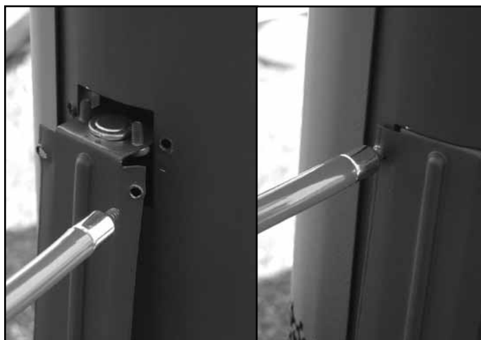
Figure 43: Spill switch installation.
