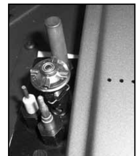
Figure 11. Ignitor assembly beside the burner.
