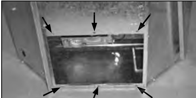
Figure 46: Removing Back Plate From Retreat.
