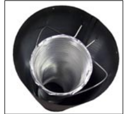
Figure 19: Wire Spacer in Place.
