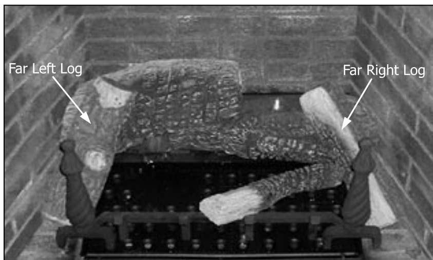
Figure 40. Third Stage Log Set Installation
