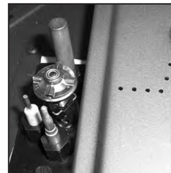
Figure 13. Ignitor assembly beside the burner.
