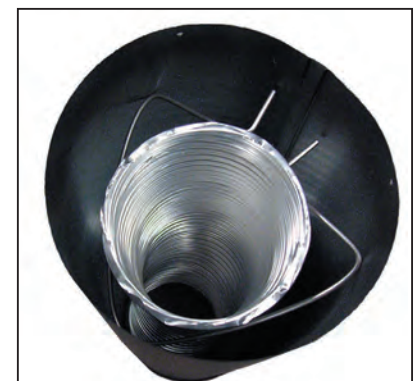
Figure 29: Wire Spacer in Place.
