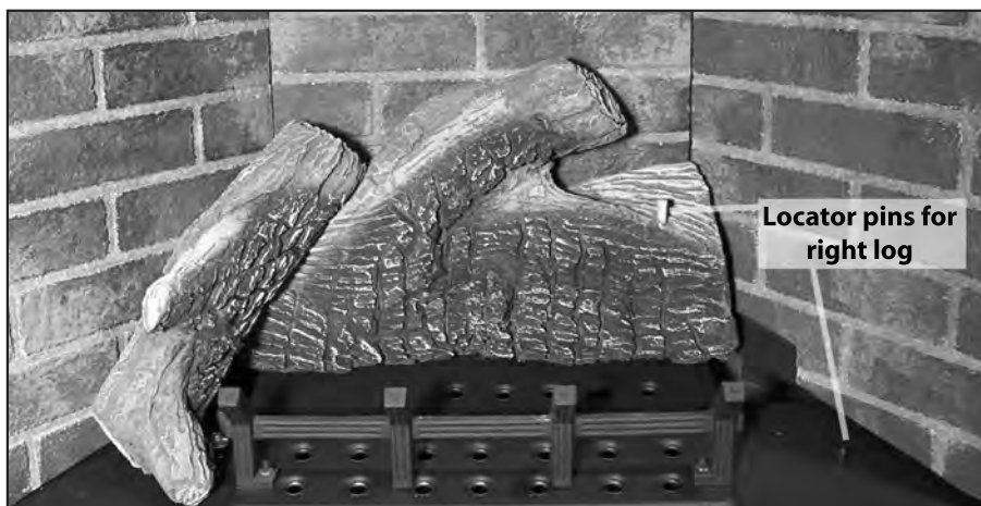
Figure 43. Second Stage Log Set Installation.
