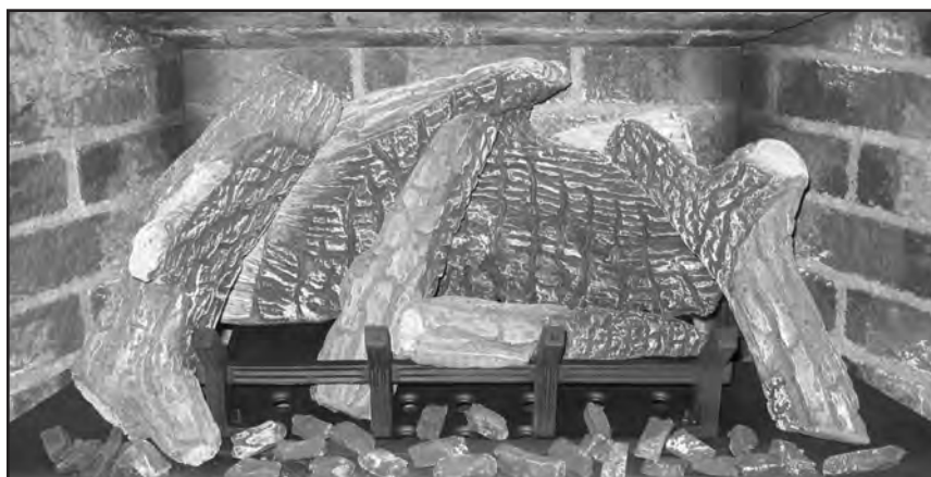
Figure 35. Fourth Stage Log Set Installation.
