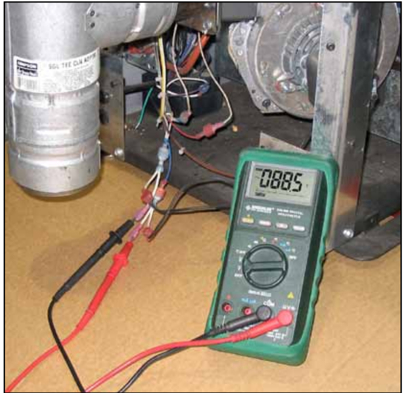
Figure 37: Measuring The Exhaust Blower Voltage.
