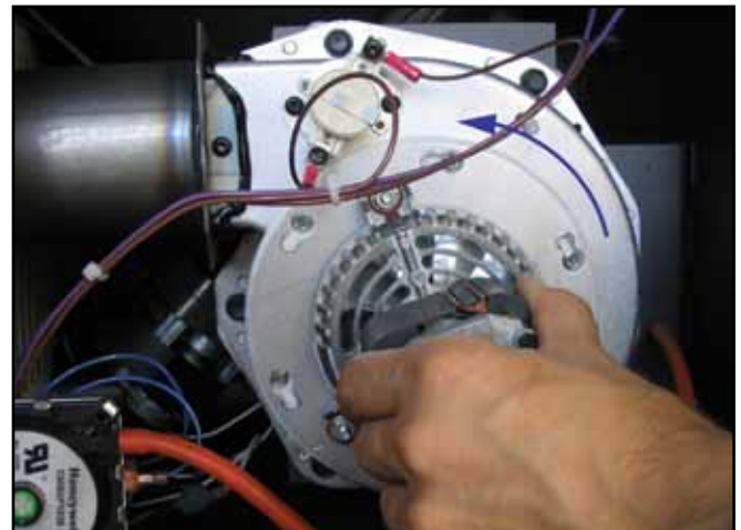
Figure 33: Removing The Exhaust Blower Motor.
