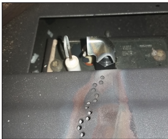
Figure 21. Correct Pilot
