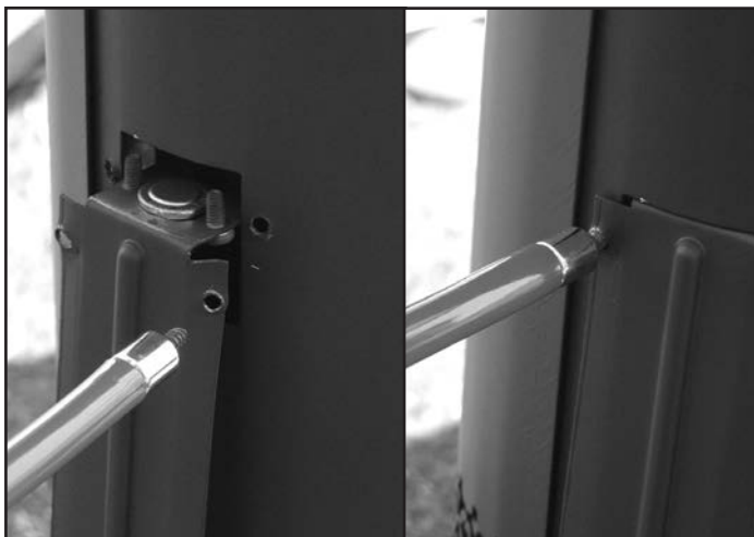
Figure 49: Spill switch installation.
