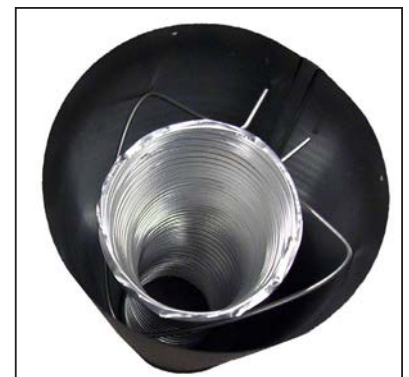
Figure 20.2: Wire Spacer in Place.
