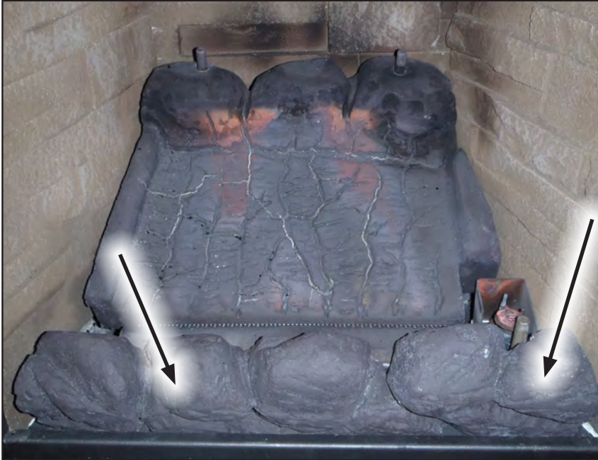
Figure 52. Second Stage Coal Set Installation.
