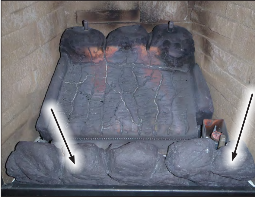
Figure 58. Second Stage Coal Set Installation.
