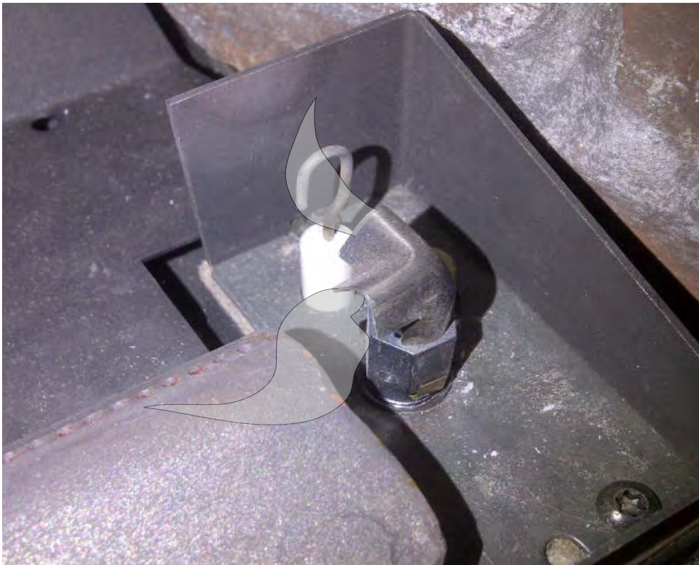
Figure 21. Correct Burner & Pilot Shield Placement
