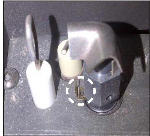
Figure 21. Pilot Slider set to LP
