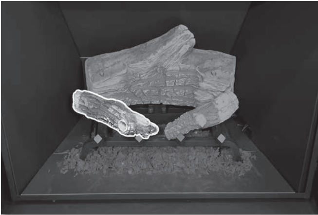
Figure 80: Log Set Installation - Step 3
