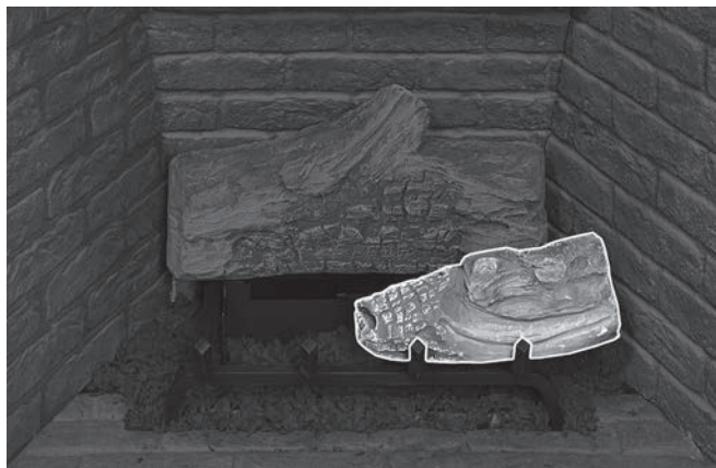
Figure 78: Log Set Installation - Step 2
