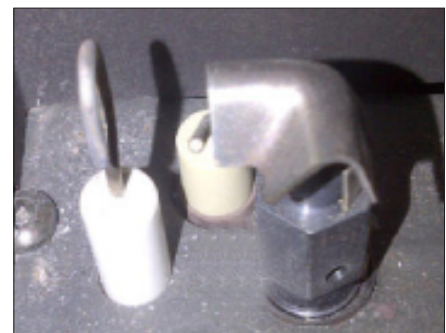
Figure 25: Correct Pilot Position
