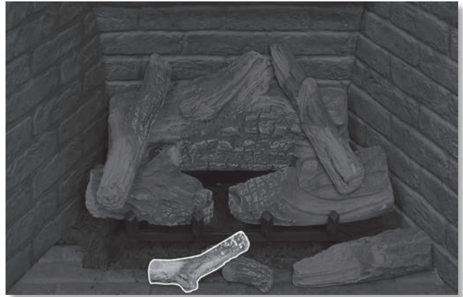
Figure 41: Log Set Installation - Step 8
