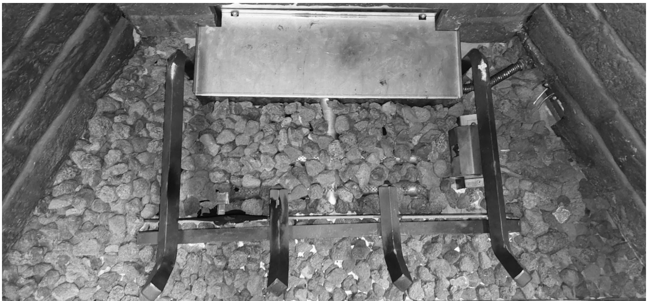
Figure 33: Lava Rock Installation
