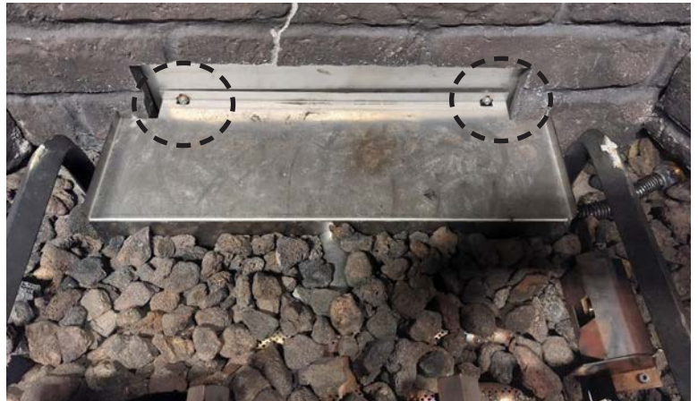
Figure 5: Venturi Cover Box Removal
